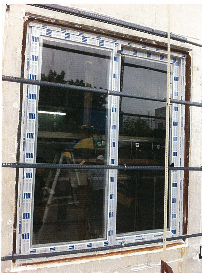
Photo 1. An exterior view of the test specimen.
